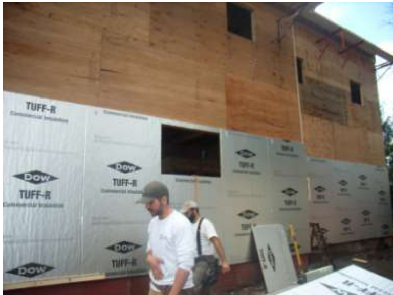
Initial layers of polyiso go up
